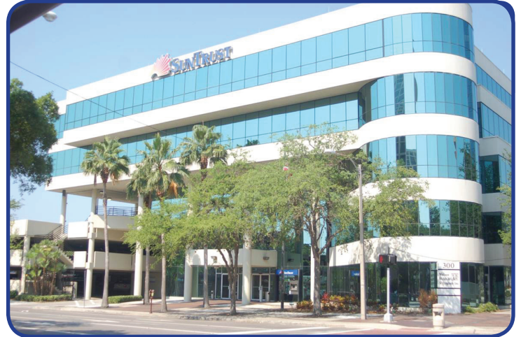
Solar Energy Management finds 40% energy reduction at SunTrust building
